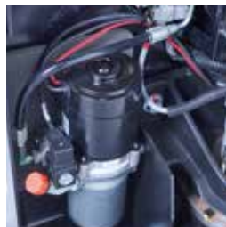
Open cell foam in motor compartment.
